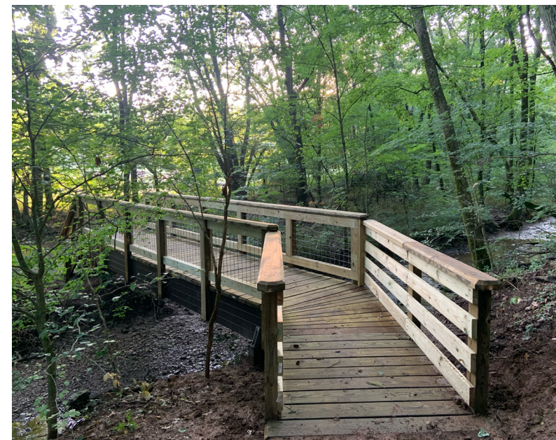
Above: Hybrid timber and fiberglass bridge in Edwin Warner Park, constructed as part of the Trail Restoration Project.
